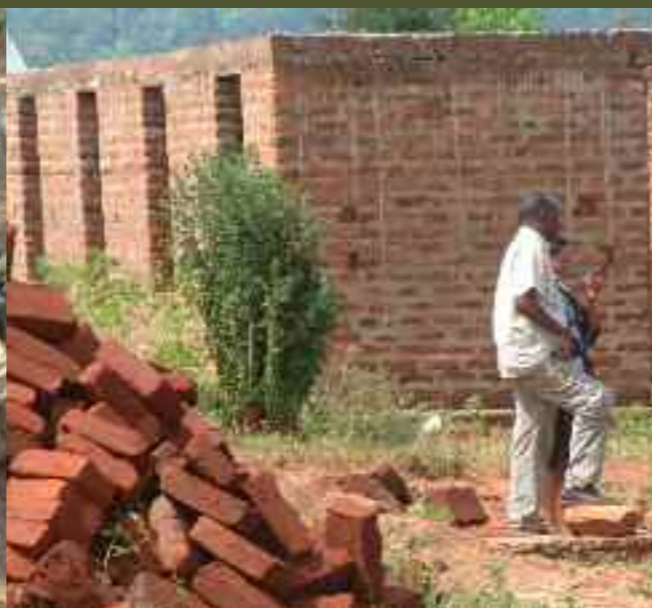
Elisaria Nnko in front of Kisiwani High School during construction
