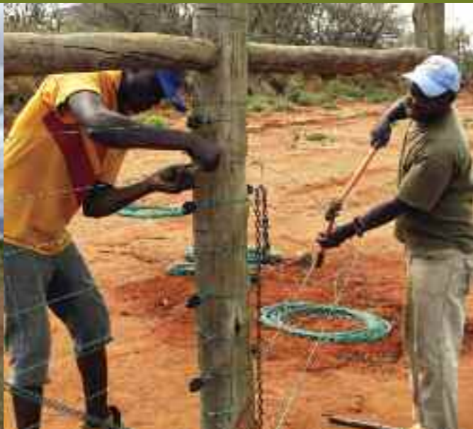
Mkomazi Rhino Sanctuary Fence Extension. Tensioning the wire.
